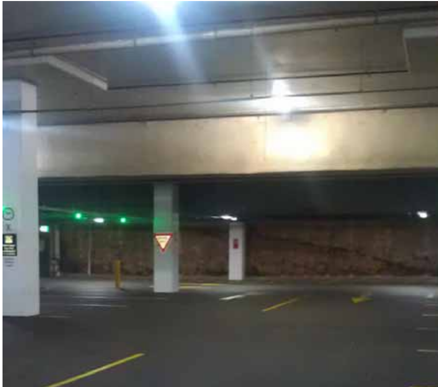
Photo 1 - Express carpark - basement cut into sandstone
